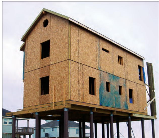
Figure 2. Construction of a Structural Insulated Panel house.
