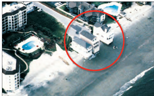
Figure 1. Well-built but poorly sited building.
