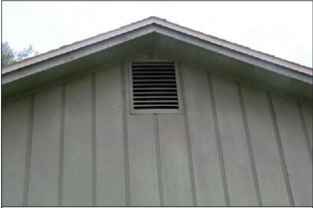
Figure 9. Gable end vent.
