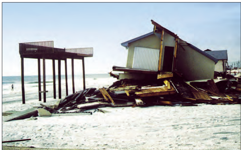
Damage from Hurricane Opal in Florida. This deck was designed to meet State of Florida Coastal Construction Control Line (CCCL) requirements. The house predated the CCCL and did not meet the requirements.
