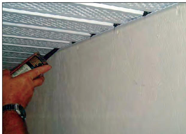
Figure 4. Applying dabs of sealant.
