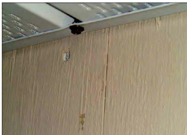
Figure 5. Screws through wall channel.
