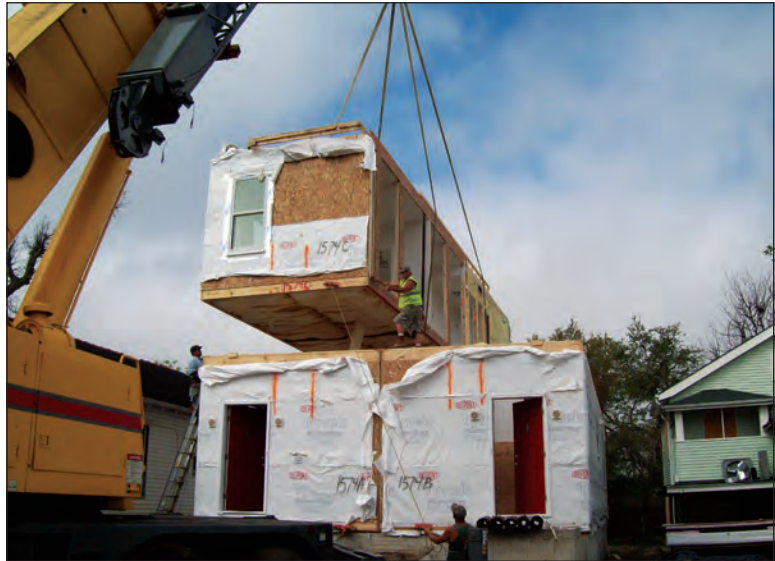
Figure 1. Construction of a modular home.
