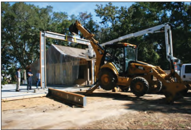
Figure 4. Installation of a prefabricated ordinary moment frame.
