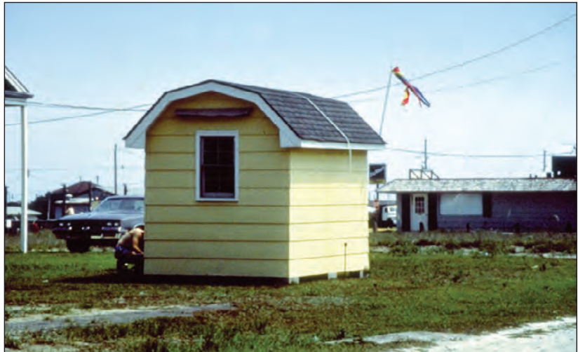
Small accessory building anchored to resist wind forces.
