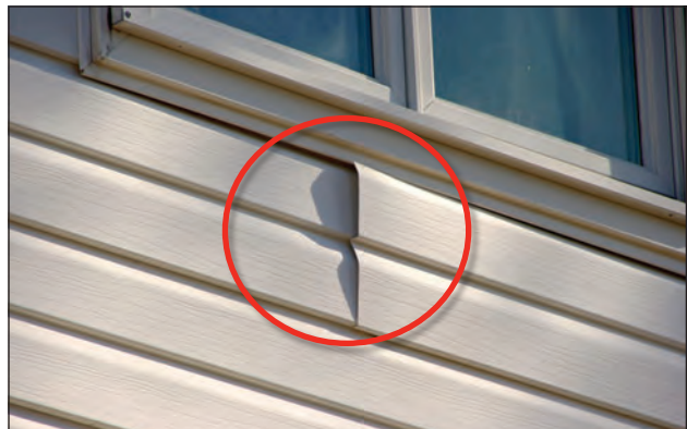
Figure 6. Proper detailing around windows and other obstacles is important. Use utility trim, punch snap-locks into siding, and do not overlap directly beneath a window.
