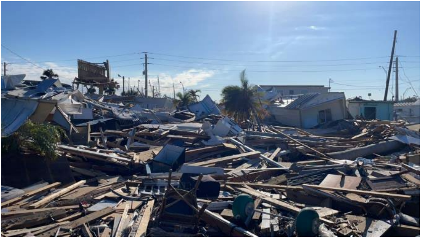
Figure 4. Damaged residential neighborhood within a SFHA located off Summerlin Road on September 29; Lee County.
