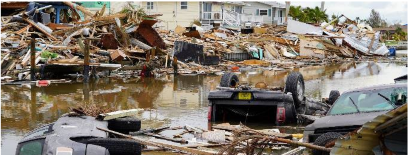
Figure 8. Photo taken of damage near San Carlos Island; Lee County.
