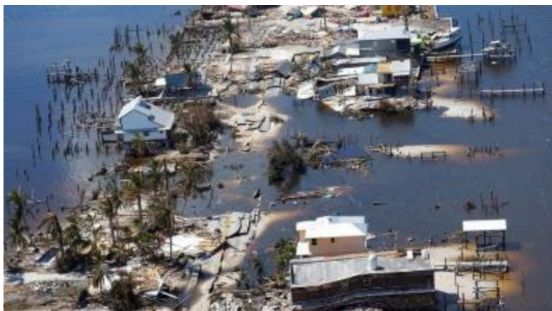
Figure 3. Matlacha Bridge damage taken on September 29; FDOT.
