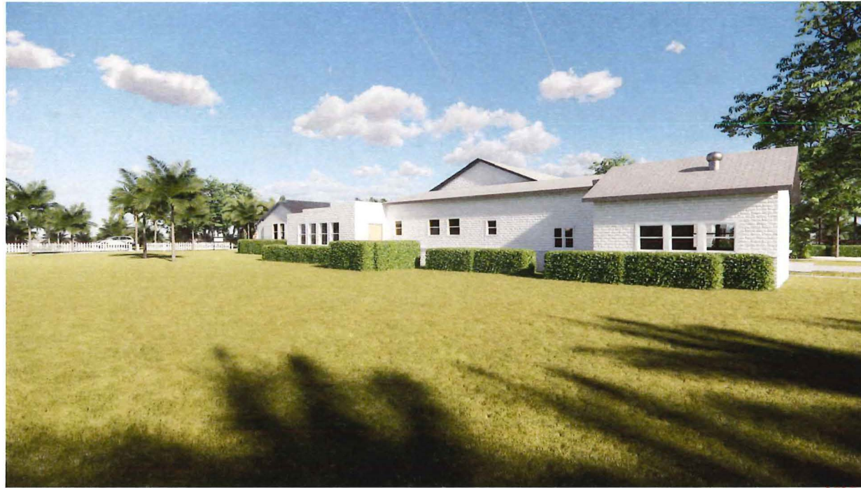
CROWNINSHEILD HOUSE EXISTING - SOUTHEAST CORNER
