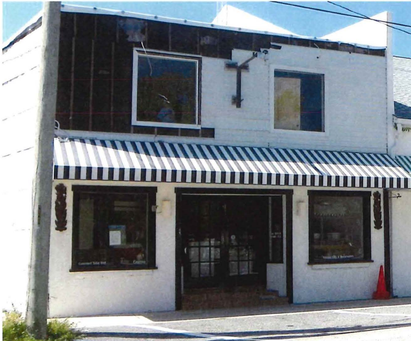
Photo of the existing awning over the sidewalk.
