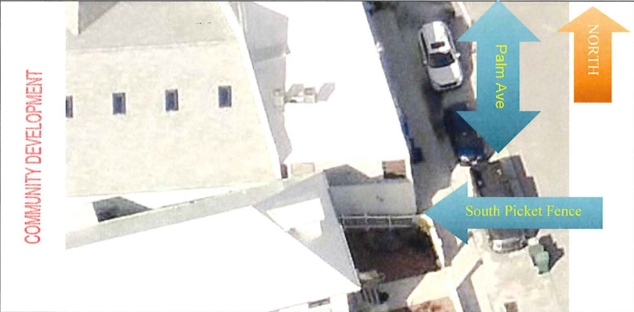
On the rear (south) is 3-ft +/- wide ramp/door landing deck providing access to the door at the rear elevation of the building. A picket fence and lattice fence separate the ramp/door landing deck from the adjoining commercial property to the south.
