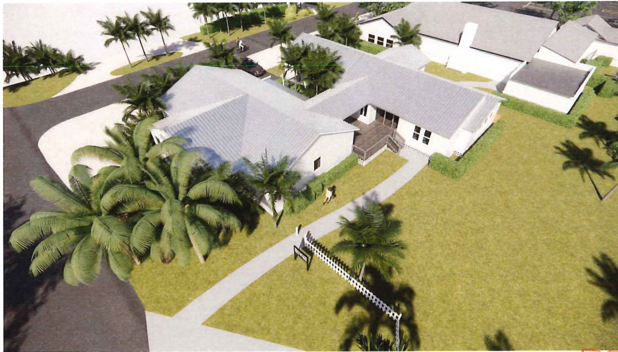
TEACHERAGE HOUSE EXISTING - SOUTHWEST AERIAL
