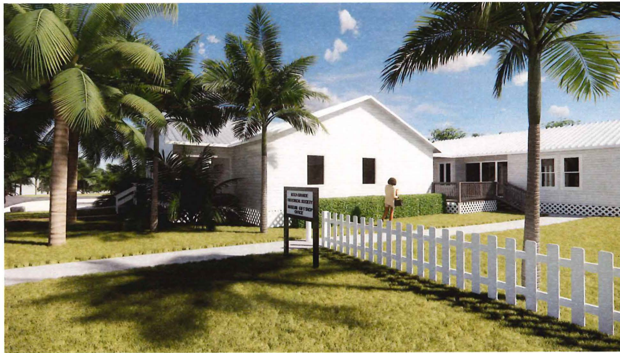
TEACHERAGE HOUSE EXISTING - SOUTHWEST CORNER
