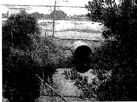
Figure 2 Drainage Canal to the east of the road. Runs under Mosquito Control property
