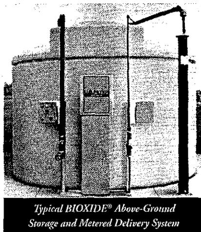
consistent dosage and lack of stability contribute to the ineffectiveness and high cost of bacteria addition. In contrast, the BIOXIDE® process provides the nutrients via a stable, easily metered aqueous solution, which promotes the growth of naturally occurring bacteria within the sewage collection system.
