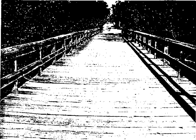
Existing wood bridge
