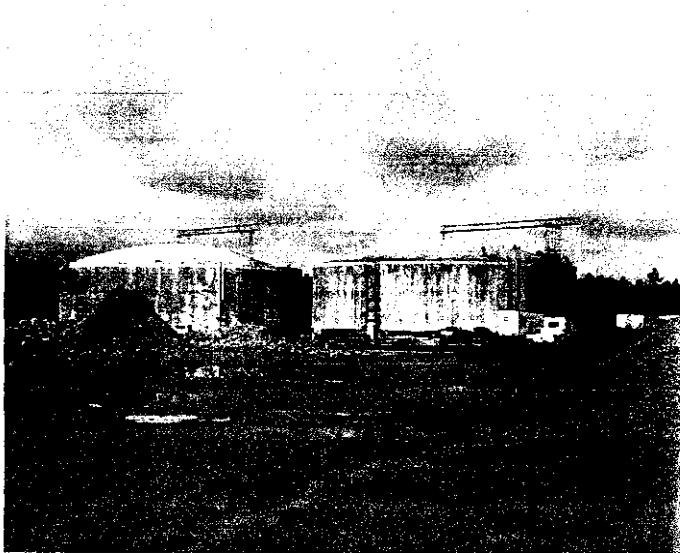
Two 5 Million gallon storage tanks to help meet the peak hour water demand from customers of Lee County Utilities.
