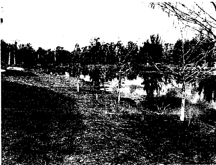
A new stormwater detention basin at Lakes Park with wetlands planting and trees along the edge.
