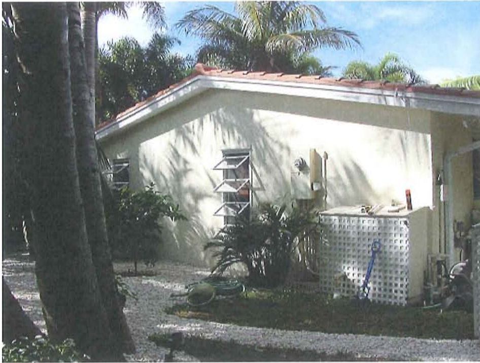
Location of the proposed addition by the Southeast corner of the house.
