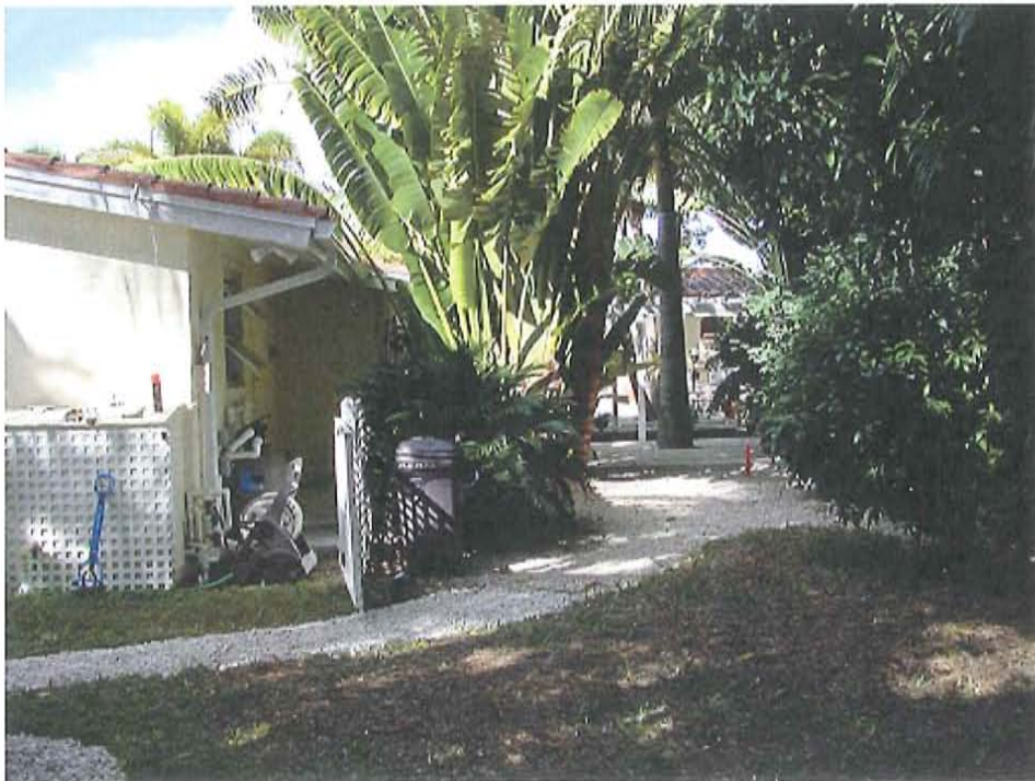
Location of the proposed addition by the Southeast corner of the house.
