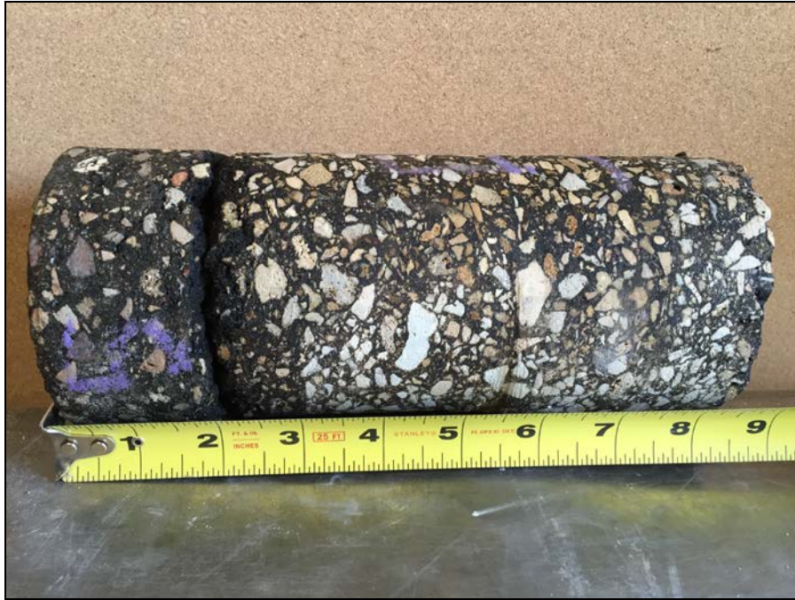
Complete debonding between Lifts 1 and 2.
