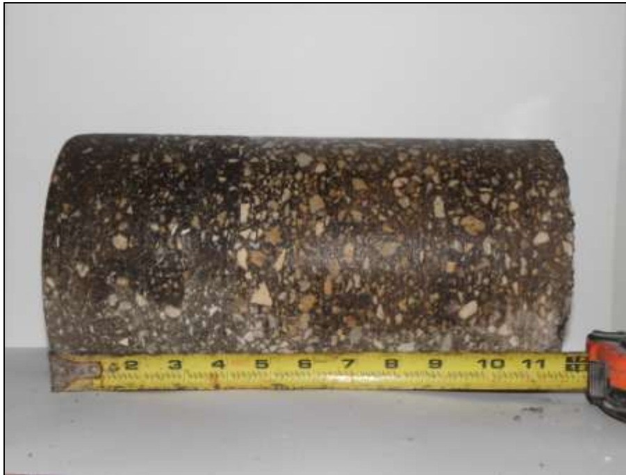
ASPHALT CORE C-3
