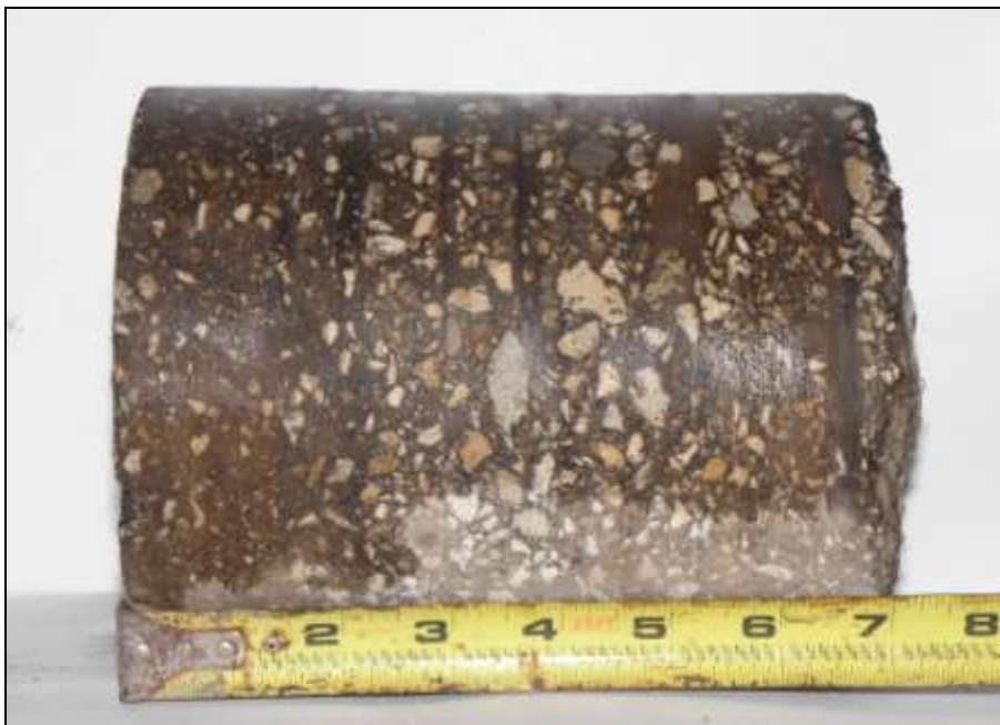
ASPHALT CORE C-4
