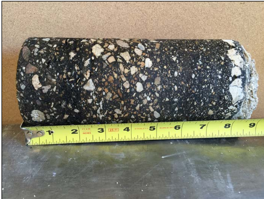
Air voids observed in Lift 2.
