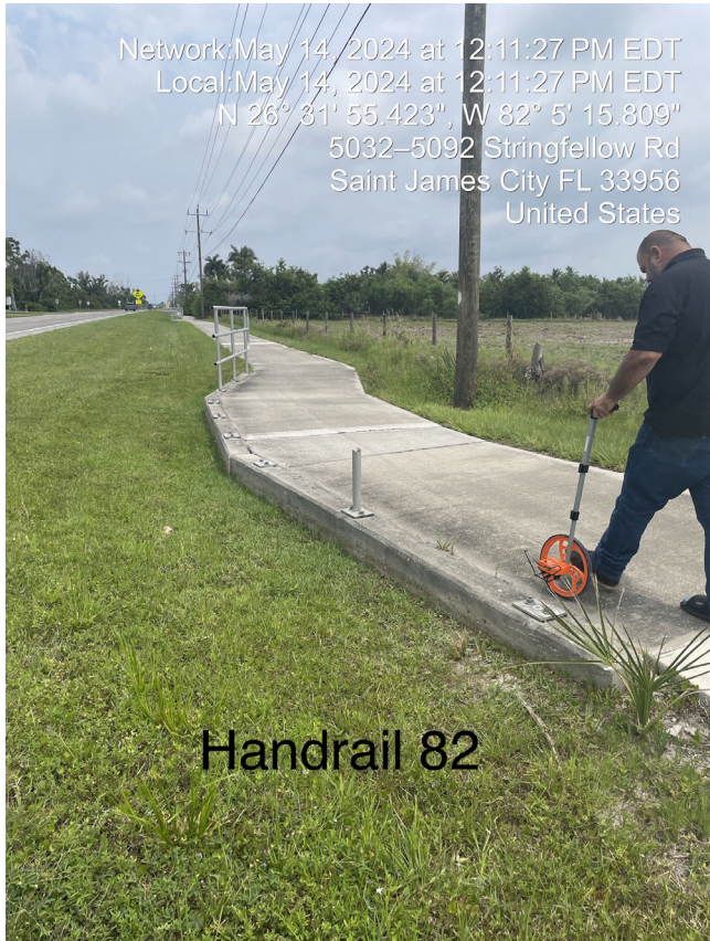
Handrail 82 Post Hurricane
