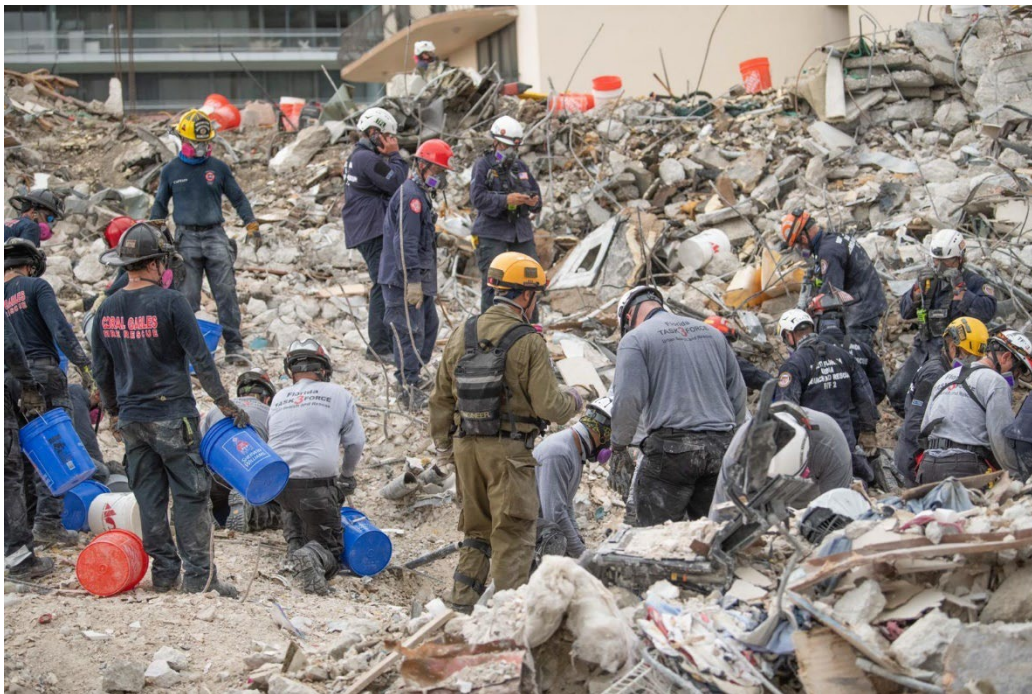
Figure 65 Surfside Condominium Collapse (2021)
