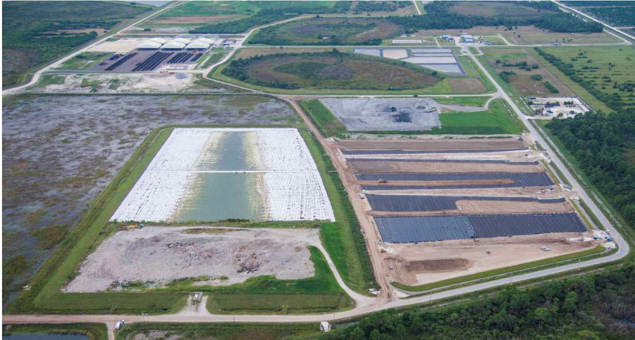
The Lee / Hendry Regional Landfill shown above includes an ash monofill, Class I and Class III landfill sites, leachate management and deep injection well, and the County's composting facility.
