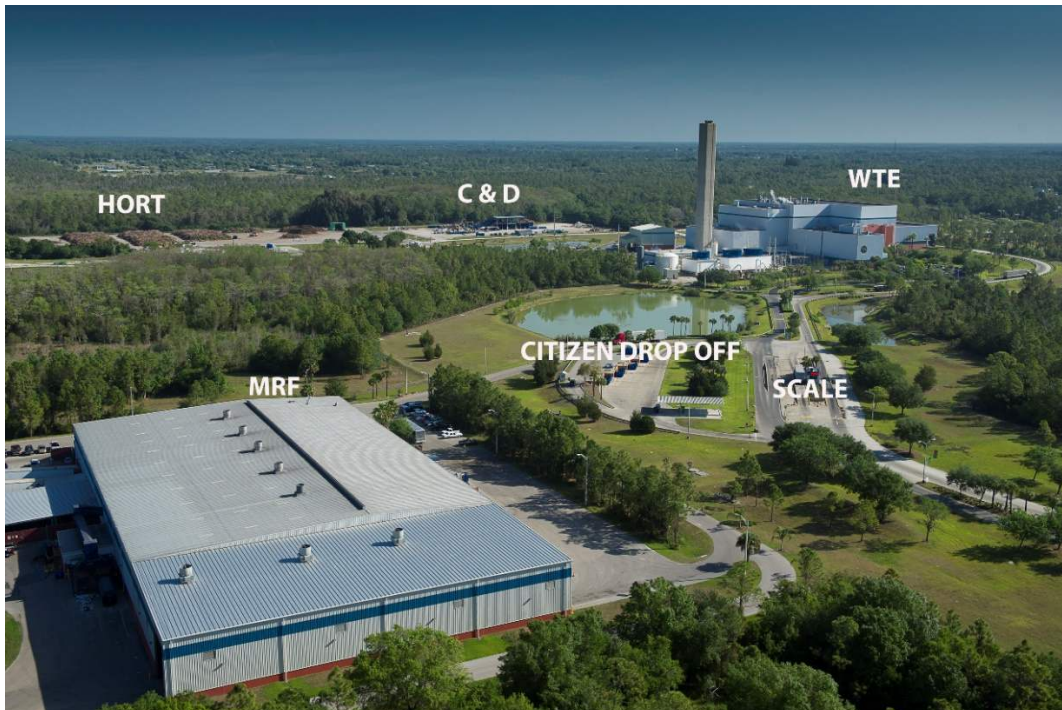
The Buckingham Campus shown above provides synergies for the integrated solid waste management system and includes the collocated WTE, MRF, C&D Recycling, MSW transfer station (not pictured), fleet maintenance, tire and yard waste processing facilities. Not shown are the County’s other disposal facilities including: Lee / Hendry Landfill, compost facility, household chemical waste, and Hendry County transfer stations.
